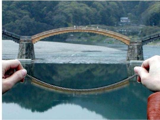
*Fig.7 Form of the arch (Catenary curve).*
